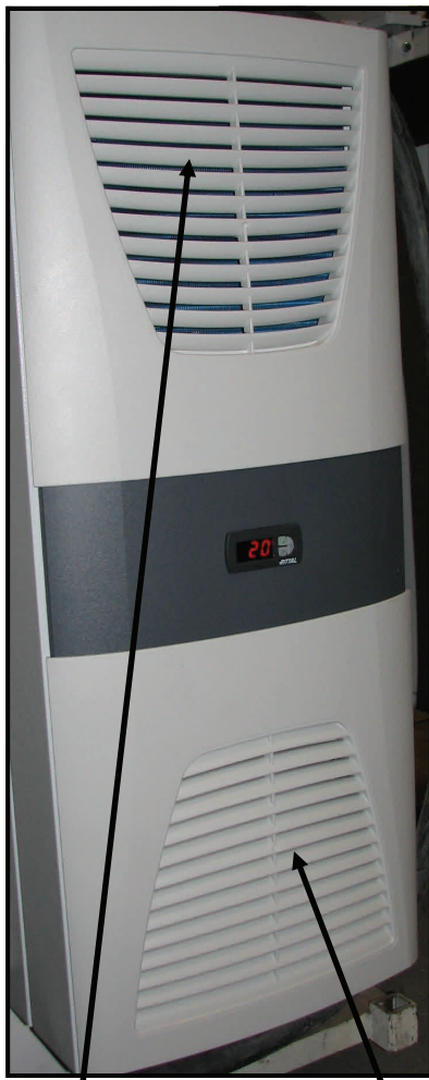
Blow out fins on the Front Cover.
