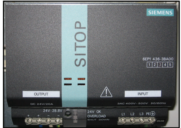
480 VAC to 24 VDC Power Supply
